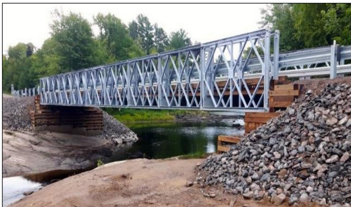
Figure 3.5: “Bailey”/ Mabey Compact Bridge
